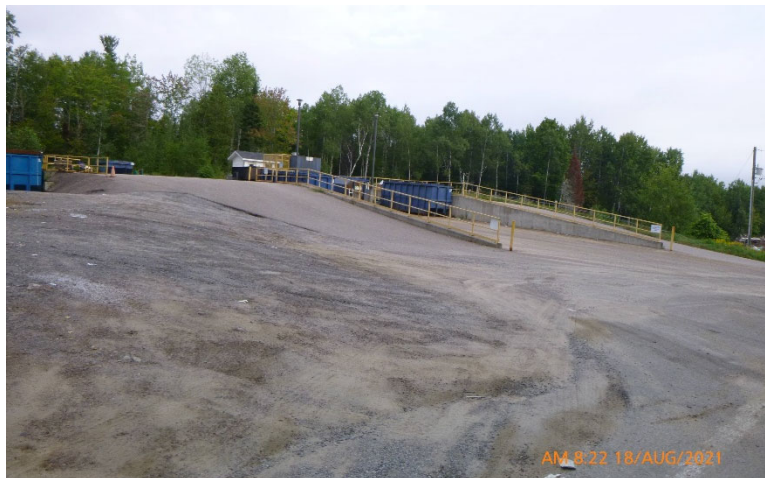
Photograph 4: Waste and Recycling Transfer Station
